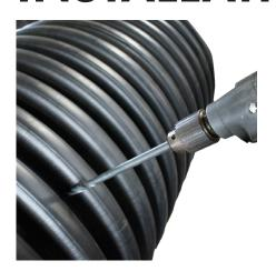
1. Use a 2 handle drill and a drill bit only, pre-drill a hole in the valley of the corrugated pipe.
