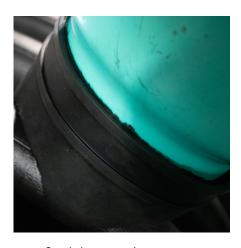
6. Insert the PVC hub into the sleeve by hand until snug. Then take a 2 x 4 and hammer to finish homing the PVC pipe into the sleeve. There are 2 tabs that will be on the inside to help ensure the pipe is fully homed.
