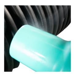
5. Once the rubber is in the hole take soapy water and spray the ID of the sleeve and the OD of the PVC hub. With your hand rub the ID of the sleeve to ensure the lube has fully applied to all areas of the ID.
