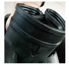
4. Grab a rubber sleeve. Fold it up with 1 alignment node facing down. Place the sleeve and the alignment node in the lower valley and begin to open the rubber sleeve to fit into the hole. Arrow should be pointing down toward pipe.
